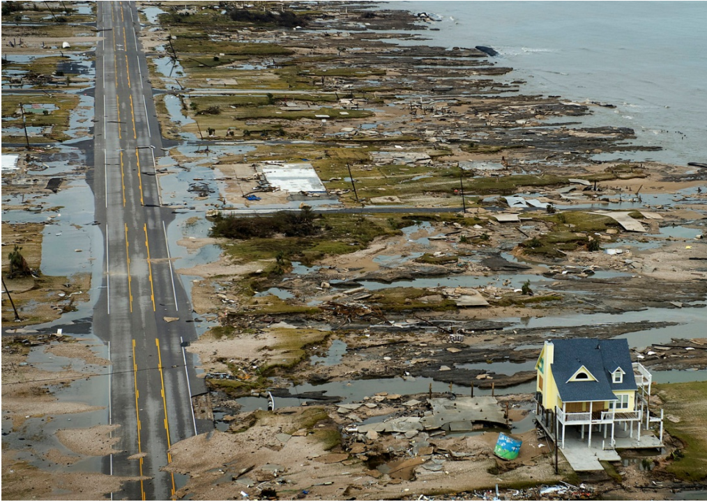
BOLIVAR PENINSULA IN TEXAS AFTER HURRICANE IKE (2008)
